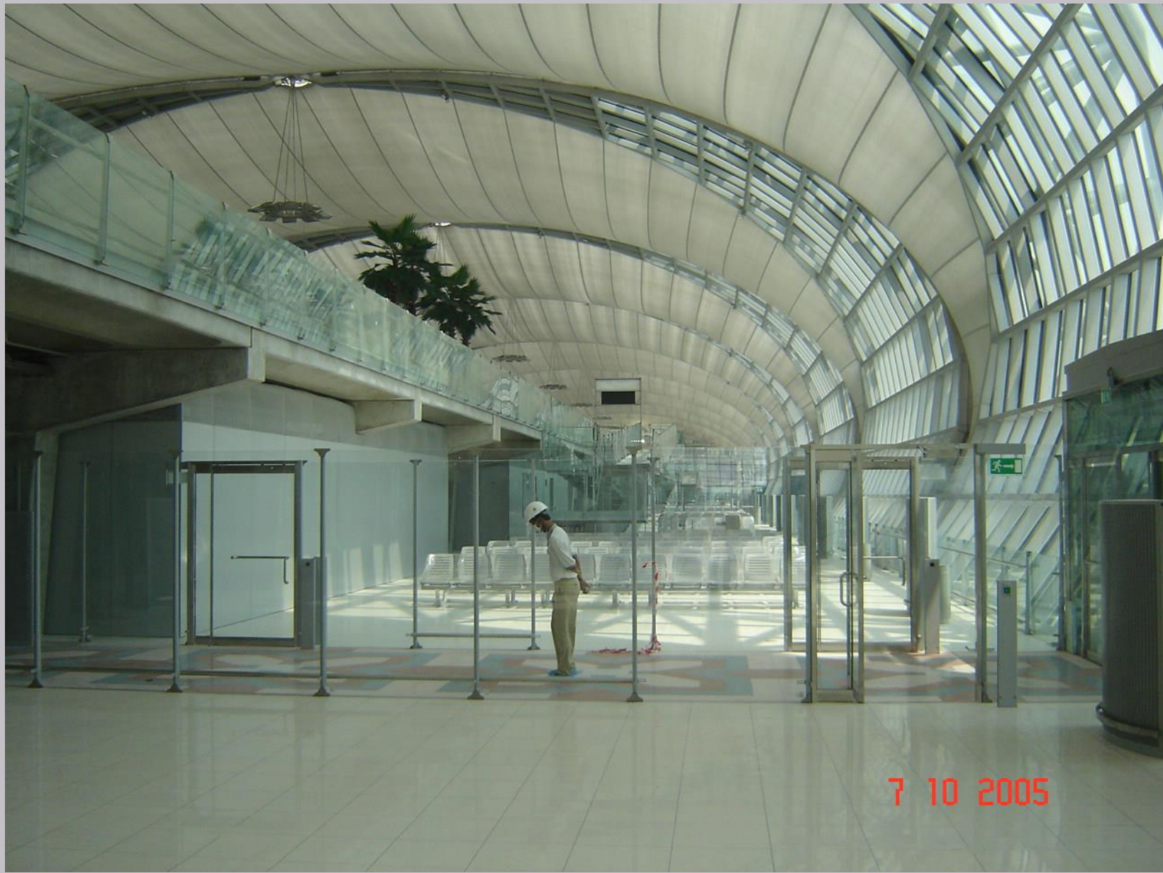
Low-e coated membrane - Bangkok International Airport, Murphy/Jahn Architects Folie 9
